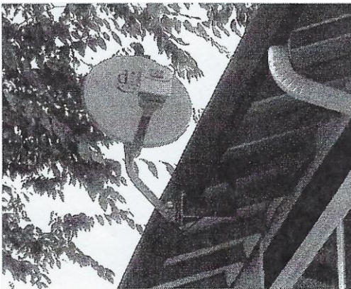
Under the eave mounting
